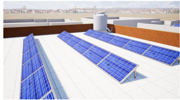
Fig. 23. Space between rows and no shadow effect (developed by researcher).
