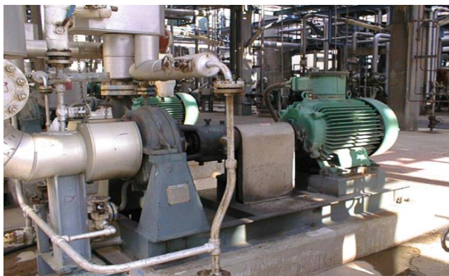
Fig. 8. Centrifugal Pump.
